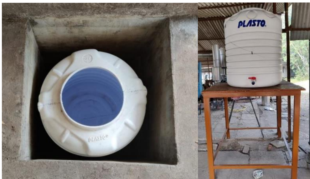
Figure 6: New collection tank (left) and settling tank (right). Figures not to scale.
