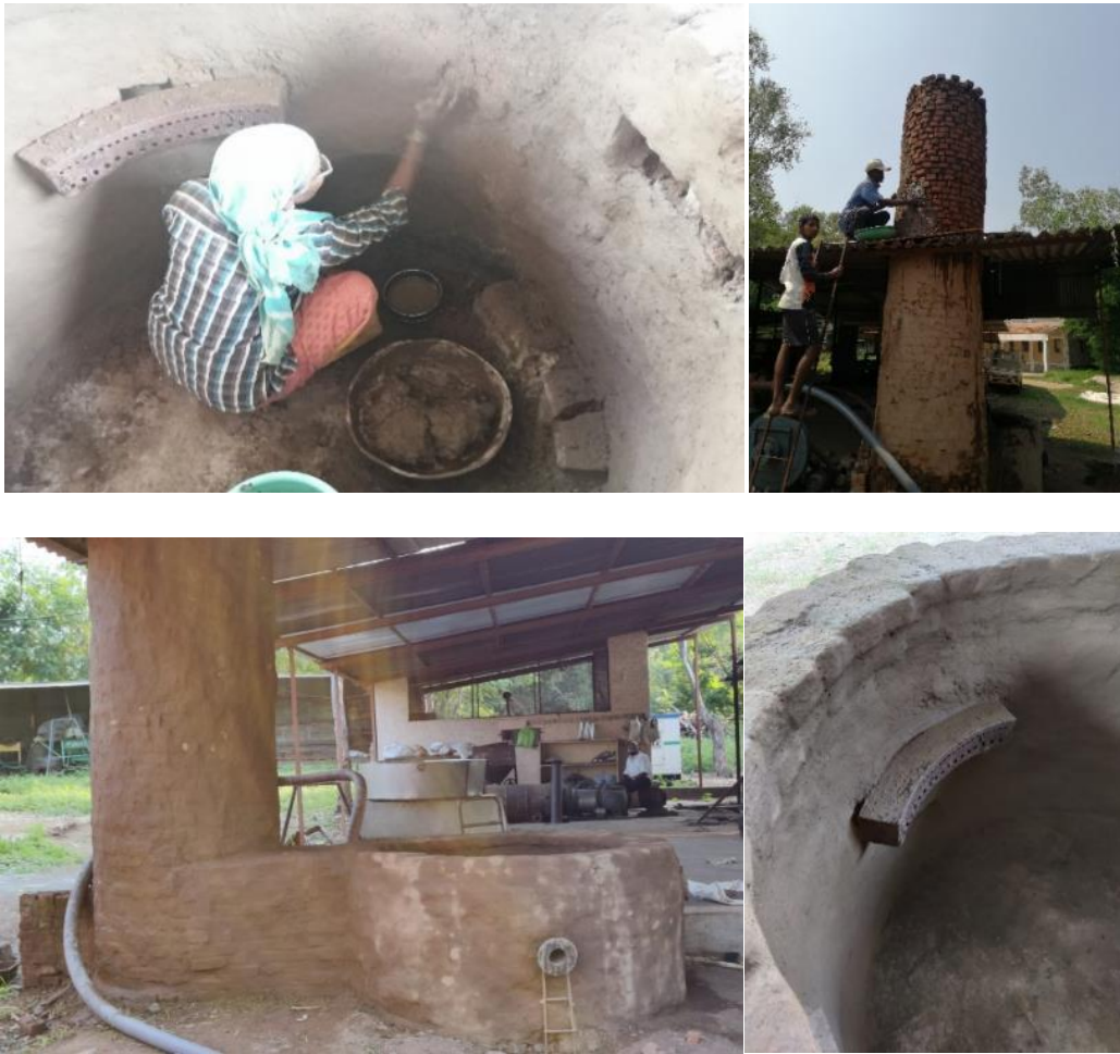
Figure 133: Reconstruction of the furnace. Top-left: plastering of the furnace; top-right: plastering of the chimney; bottom-left: renovated furnace; bottom right: blower connection.
