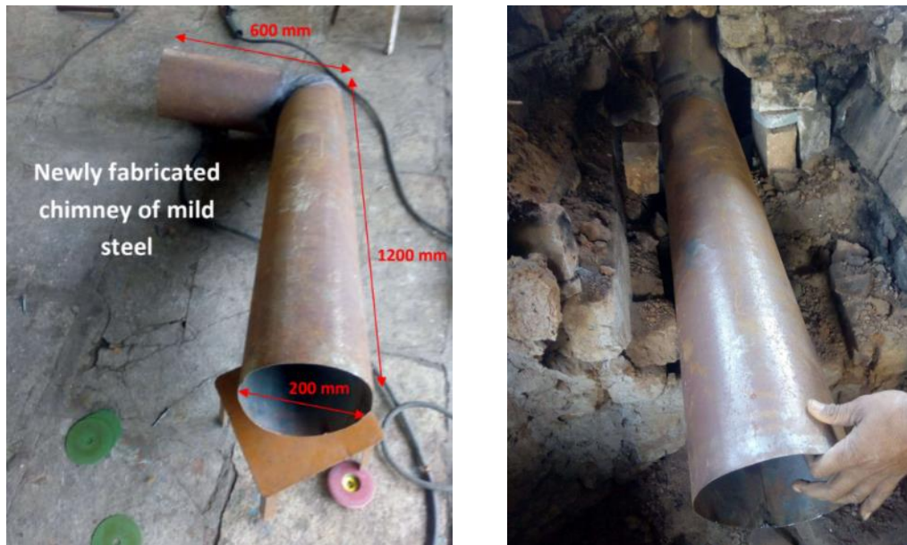
Figure 143: L-shaped chimney. Left: before assembly. Right: during assembly.
