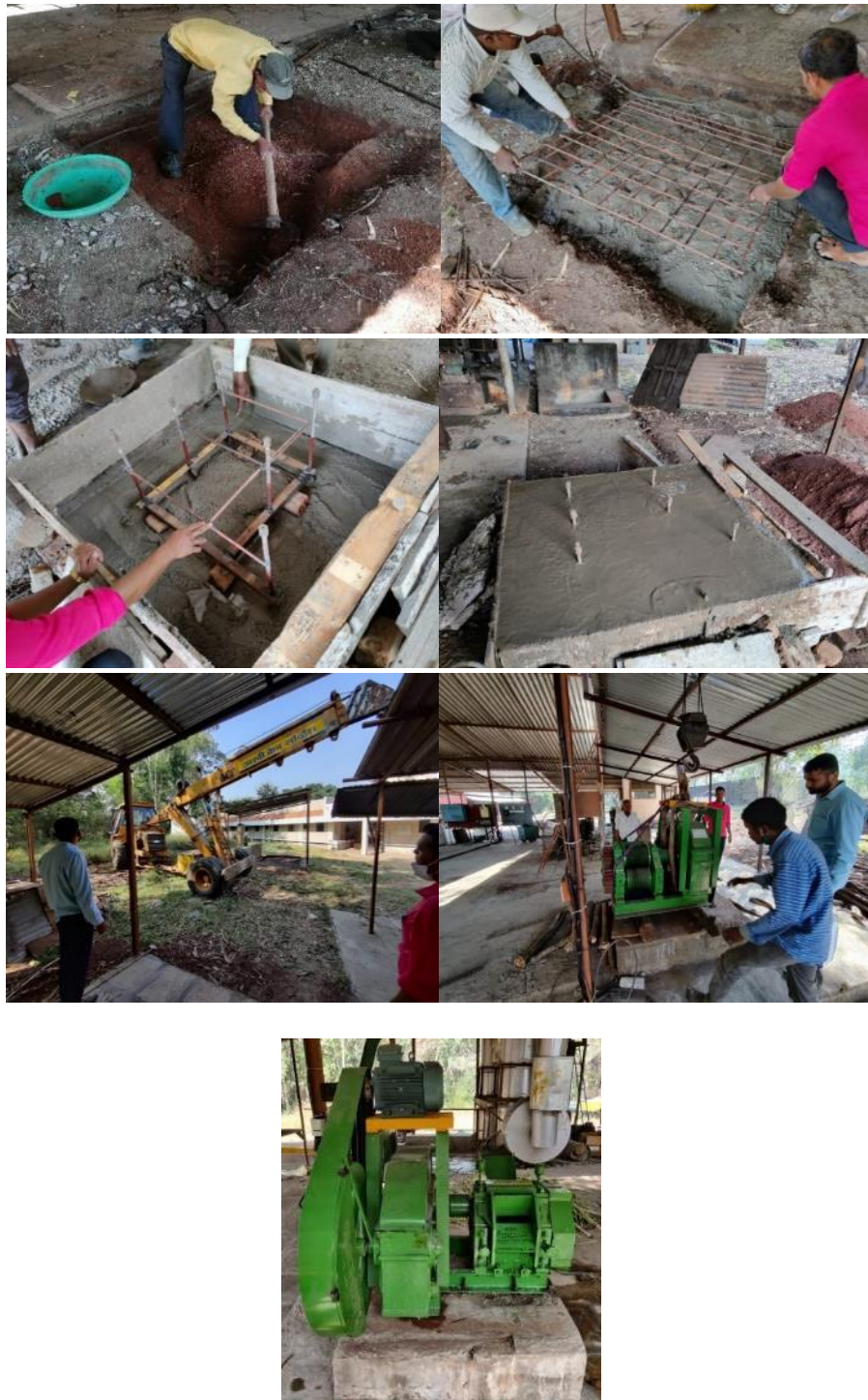
Figure 104: Work from foundation construction to crusher installation.
