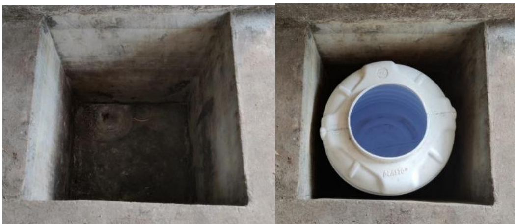
Figure 35: Left: previously used 650 L cement collection tank; right: new 300 L plastic collection tank.
