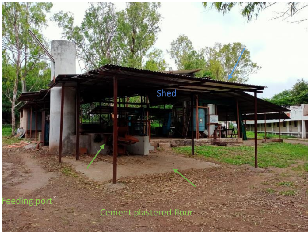
Figure 74: Area in front of the feeding port was plastered with cement.
