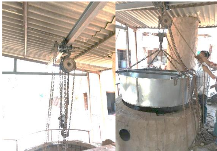
Figure 122: Installation and trials on old chain block.
