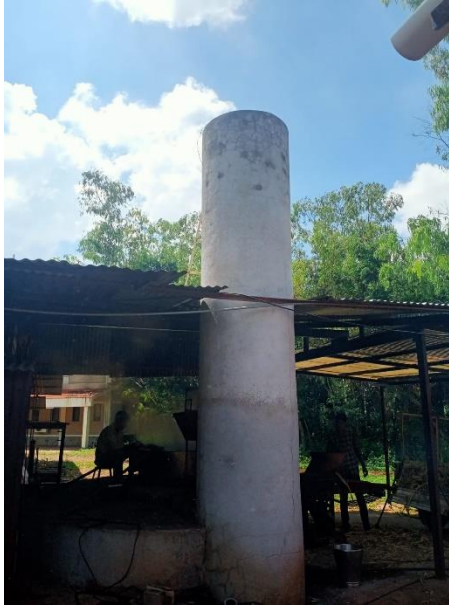
Figure 14: View of the chimney during a syrup-making session. The outgoing smoke through the chimney is transparent, indicating clean combustion.
