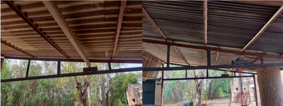
Figure 121: Structure erected for installation of block and tackle.
