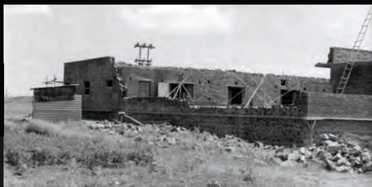
NARI main building under construction, 1979
