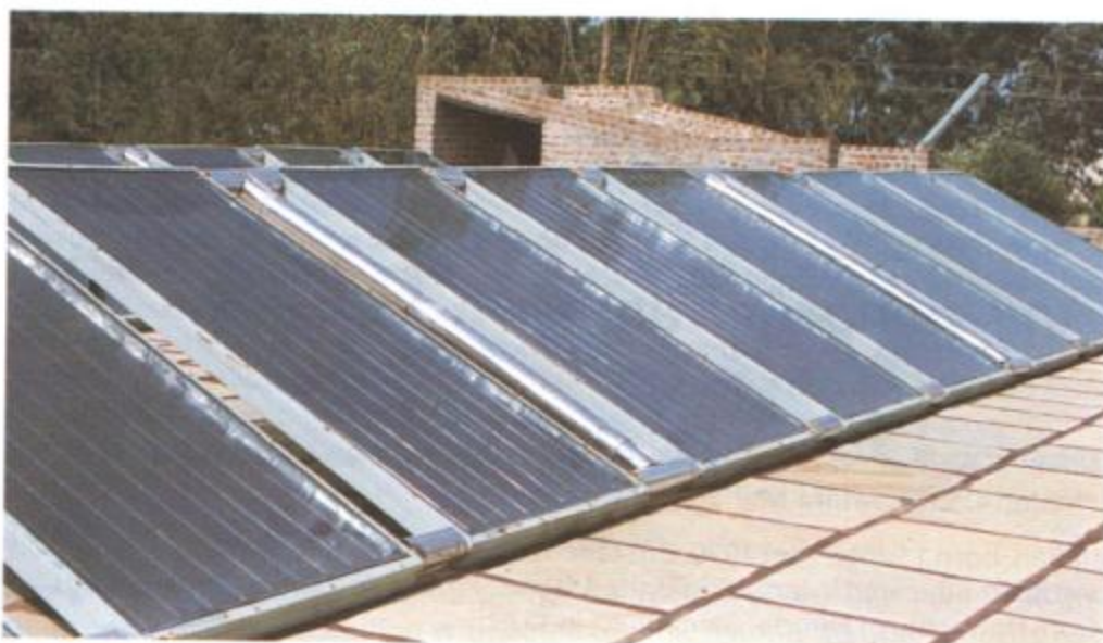
Alcohol distillation plant running on solar energy capable of producing 30–150 litres/day 95% (v/v) ethanol. On the right is shown the solar hot-water storage tank.
